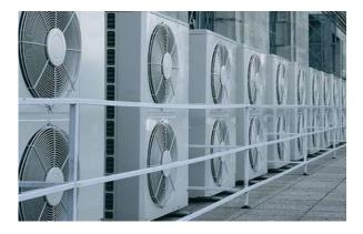
For the condensation of refrigerants in commercial and industrial refrigeration systems.
